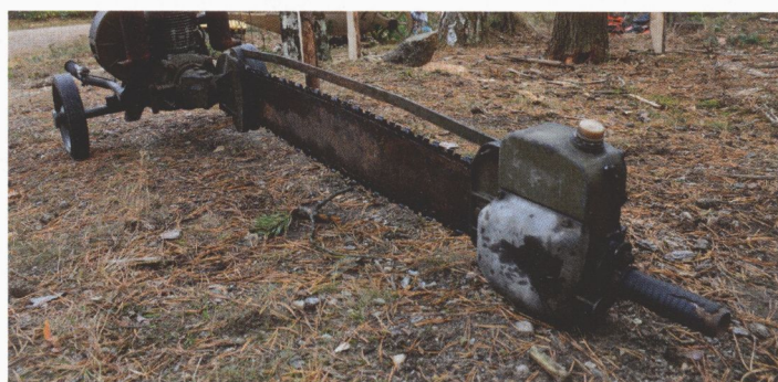
The first chainsaws used in logging were operated by two men. They were so heavy, wheels were needed to transport them.
