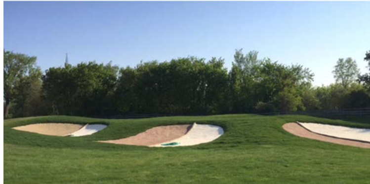
Construction (top) and final product (bottom) of the LGD Bunker Laboratory where we've pitted various liners and sands against each other. Despite a wet summer, we have yet to do more than hand rake animal footprints!
