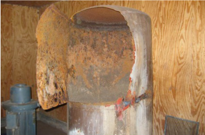
Tanks are pressurized with compressed air and can explode.
