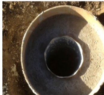
The flag pole sits in a sleeve that allows it to be straightened if it begins to lean over time..
