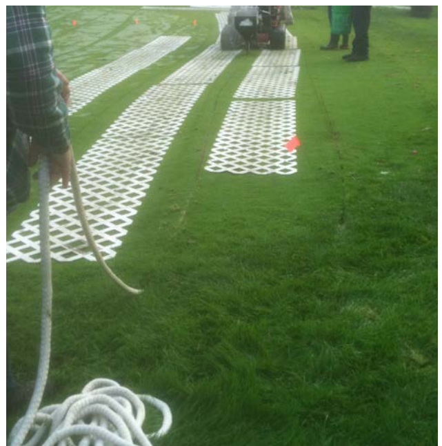
A vibratory plow is used to install the drainage element into the soil with minimal disruption to the surface.
