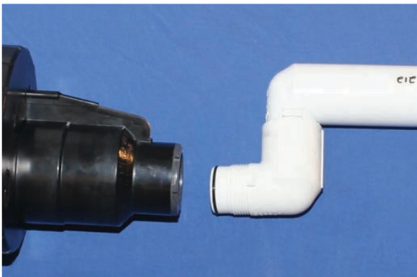
Figure 3. ACME outlet on swing joint (note o ring that identifies the male threads as ACME)
