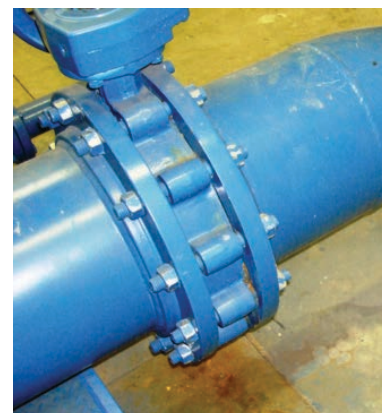
Figure 1. A bolt through flanged valve.
