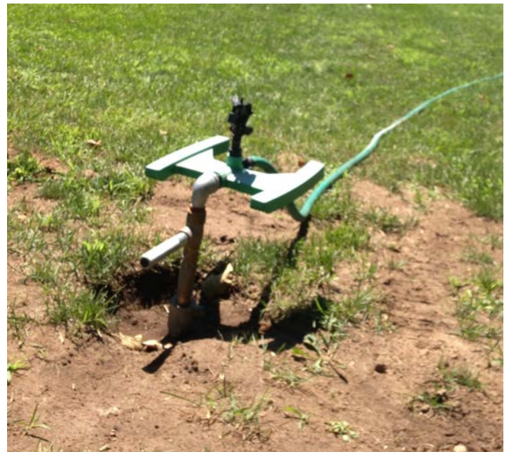
A problem solved with a little ingenuity and a trip to the local hardware store.
