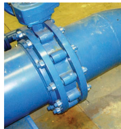
Figure 1. A bolt through flanged valve.
