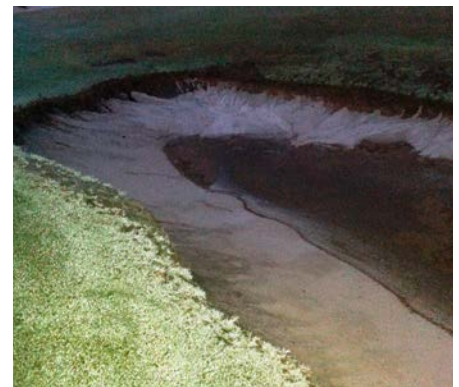
One of the bunkers that needed some sand pushed back into place after the rainfall event on Thursday night.
