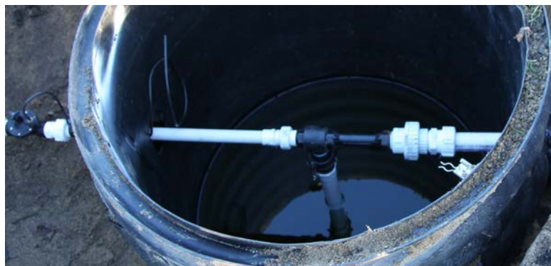
One of the Irrigation Drive Pumps (IDPs) in the early stages of installation in a sump. They sound more complicated than they really are.
