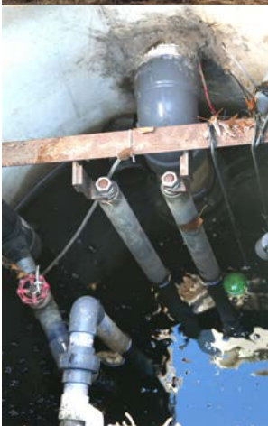
One of the main 10' concrete sumps being installed housing the main 7.5 HP pump that moves most of the water off the property. The switch that actuates the pump is triggered by the weight of the water within the sump.
