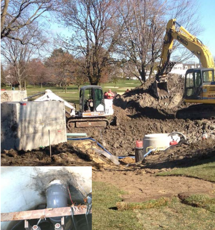
One of the main 10' concrete sumps being installed housing the main 7.5 HP pump that moves most of the water off the property. The switch that actuates the pump is triggered by the weight of the water within the sump.
