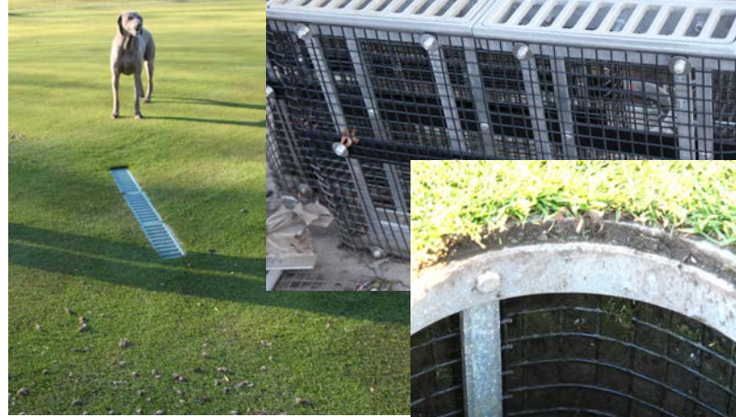
When drains vent to the surface grates are held in place by metal cages wrapped in fabric allow air and water exchange from the surrounding soil too.
