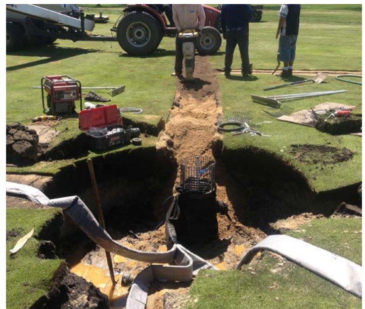
The Leibold construction crew compacting sand in one of the trenches.
