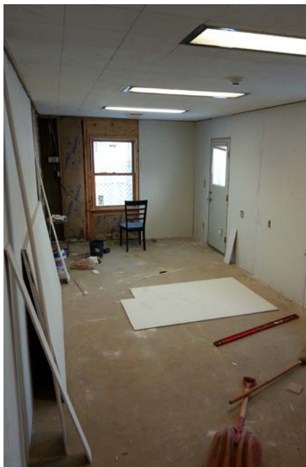
The new drywall took a day to hang.
