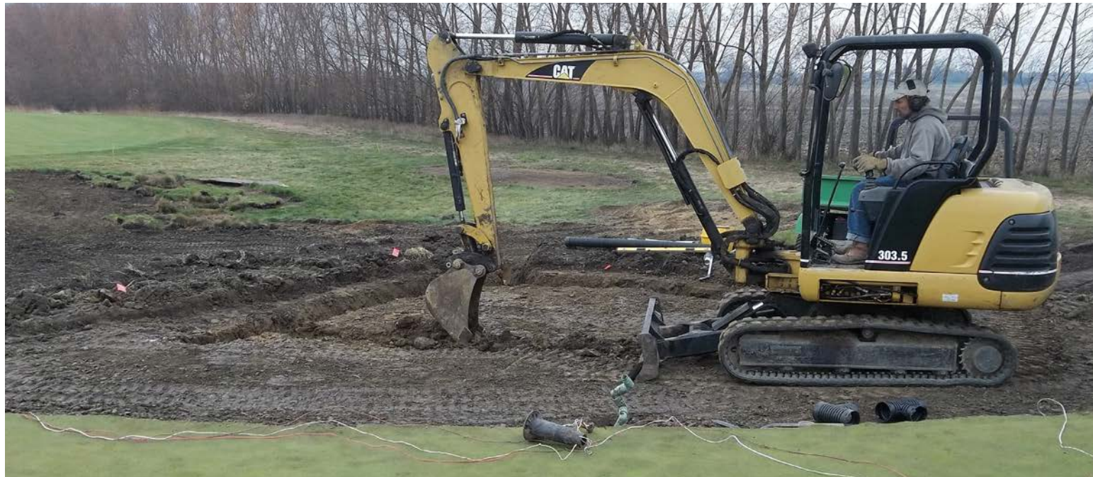
Mike Reardon begins to cut drainage trenches to tie the new part of the green into the existing drain lines.
