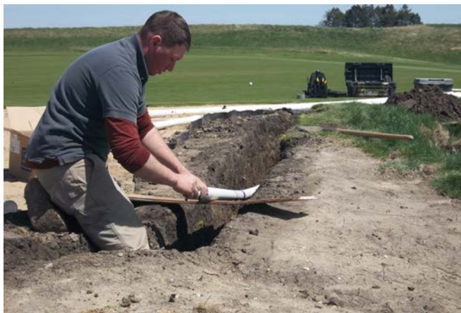
After measuring proper irrigation head spacing, the staff re-routes lines and places piping for each head.
