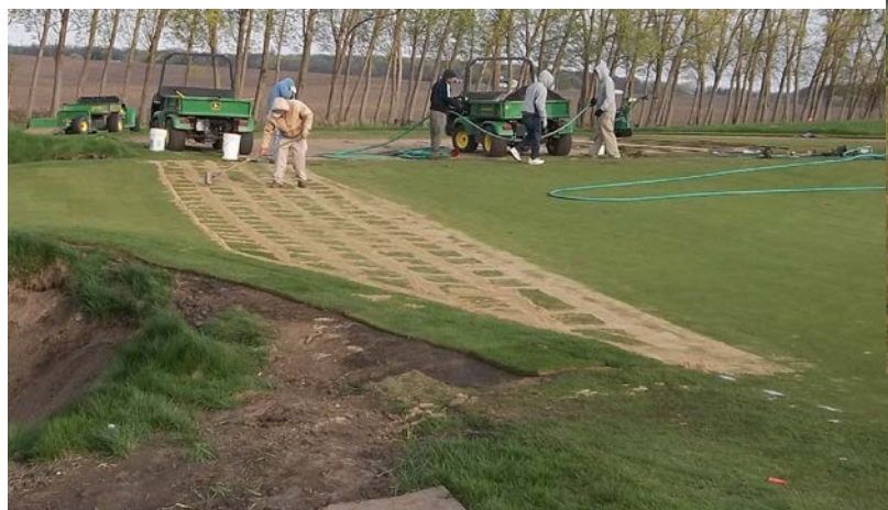
Black Sheep staff topdressing seams on new sod and preparing new bunkers for liner installation during the early spring of the year.
