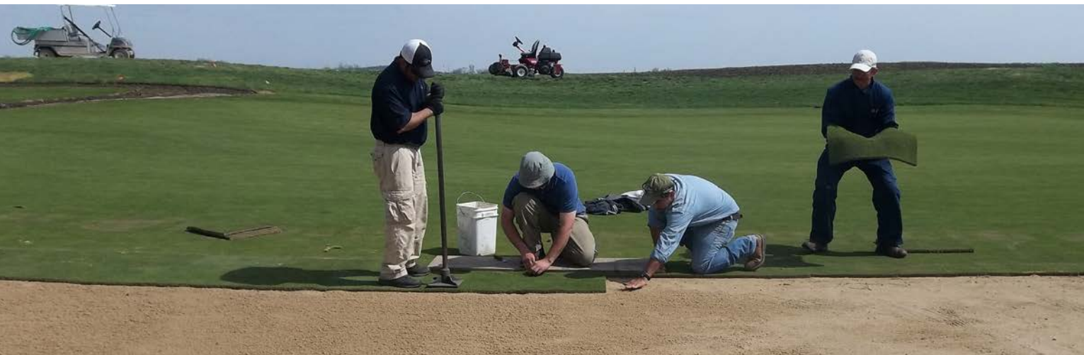
Staff carefully moves sod from existing section of the green to the new portion. Green was constructed using the California method of putting green construction.
