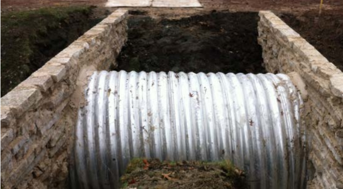
After the pipe was set in the ditch and footers were poured, skilled staff members at Indian Hill Club began the stonework.
