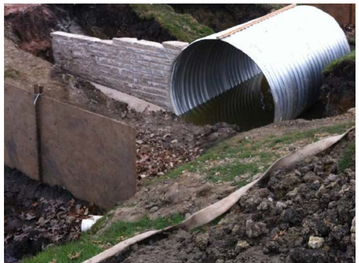
The plywood in the forefront was used to temporarily damn the water. As the water rose, pumps were used to transfer water to the low side of the ditch.
