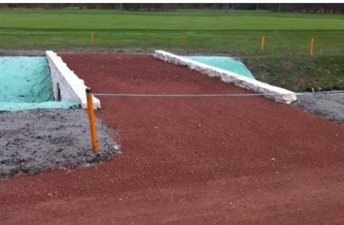
After each bridge complete and backfilled, staff finished off the grade with crushed red stone to match the existing path work at IHC.
