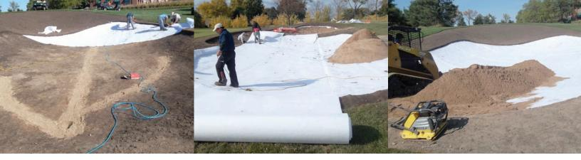
At this point all the drainage lines were exposed, so the next step was to remove all the p-stone and discard it with the old sand. Then the drainage pipe was disconnected and brought outside of the bunker to be cleaned thoroughly. We also wanted to make sure that all the drainage lines leaving the bunkers were draining properly so they were flushed with water. Once they were certain that everything was working, the pipe was placed back into the trenches and backfilled with new p-stone.
