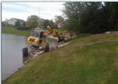
Low Impact Construction Methods
