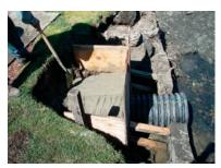
After the rain, we needed to dig around the pipe again to prepare for more concrete to seal the pipe to the concrete tank and to hold the pipe in place. **•OC**
