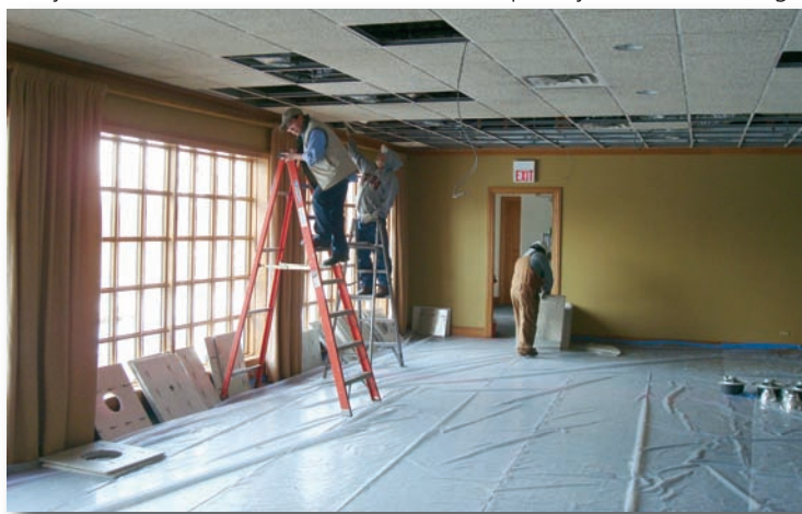
Members of the grounds staff install new drop ceilings in the dining rooms this winter. It saved on the cost of the project and allowed Tim to keep staff members throughout the winter months.
