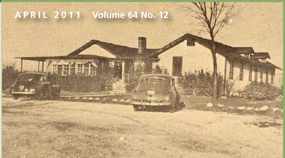
Naperville's clubhouse and "Porch" the way it used to be.
