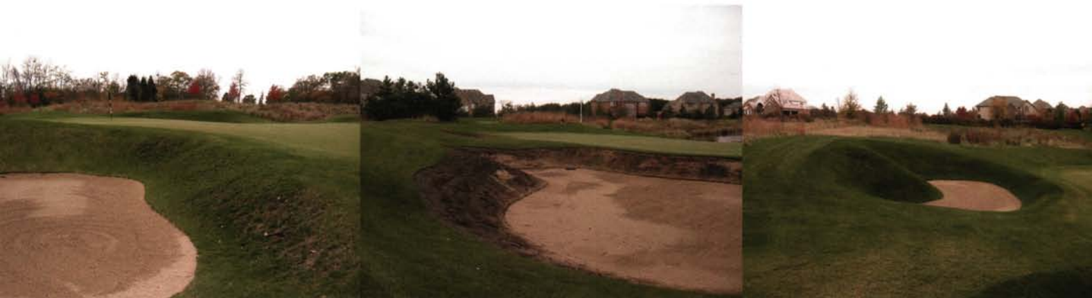
From Left to Right: The steep sloping embankments with struggling bluegrass, a bunker with the slopes prepped for sod, and a completed bunker embankment planted with new low mow cultivars of Kentucky bluegrass.
