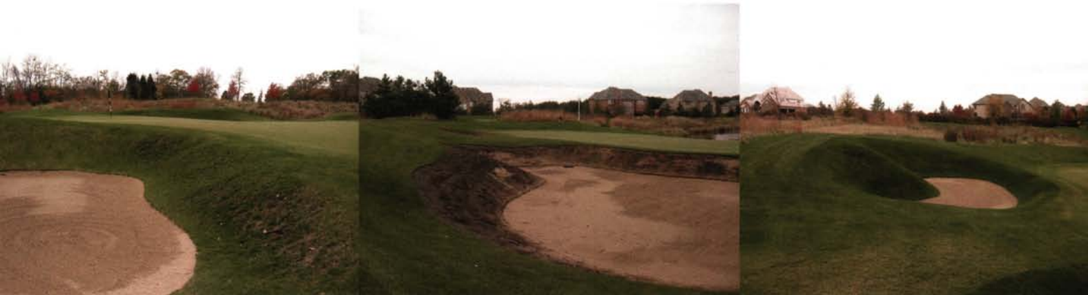
From Left to Right: The steep sloping embankments with struggling bluegrass, a bunker with the slopes prepped for sod, and a completed bunker embankment planted with new low mow cultivars of Kentucky bluegrass.
