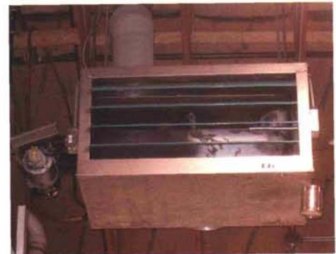
The new waste oil heater. Waste oil is pumped to the heater through the copper tubing to the left.
