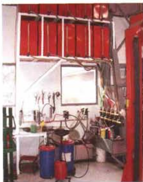
Biltmore's oil supply system—storage tanks above, valves to the right, and waste oil tank below.
