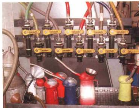
Notice the color coding of each filling can and hose on the valve panel.
