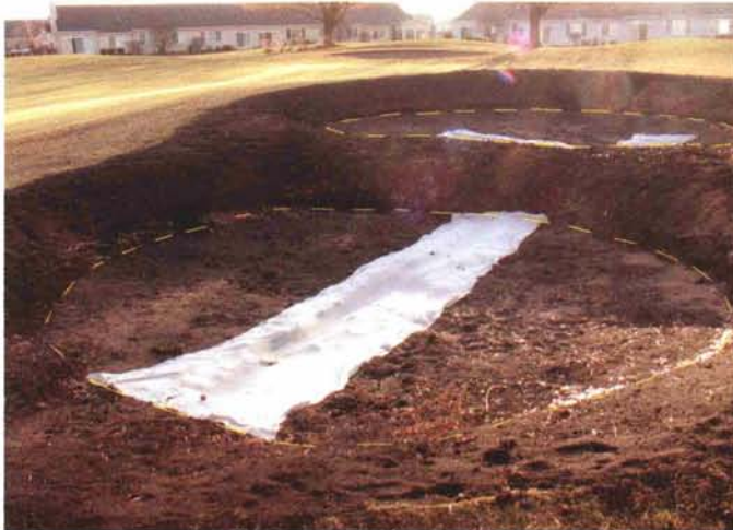
Bunkers on the Blue Course No 6 Green ready for sand.
