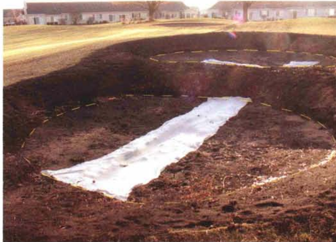
Bunkers on the Blue Course No 6 Green ready for sand.
