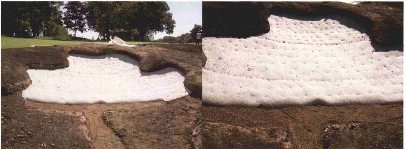
Sandtrapper II liners were used in cases where sand-flashing slopes presented erosion potential; liners were tucked into the drainage mechanism.
