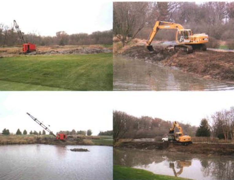
The dredging of the watershed and the grading of the shoreline at Rich Harvest Farms number seven.
