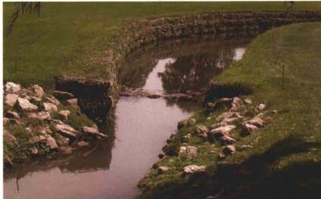
An example of erosion control for stream banks.
