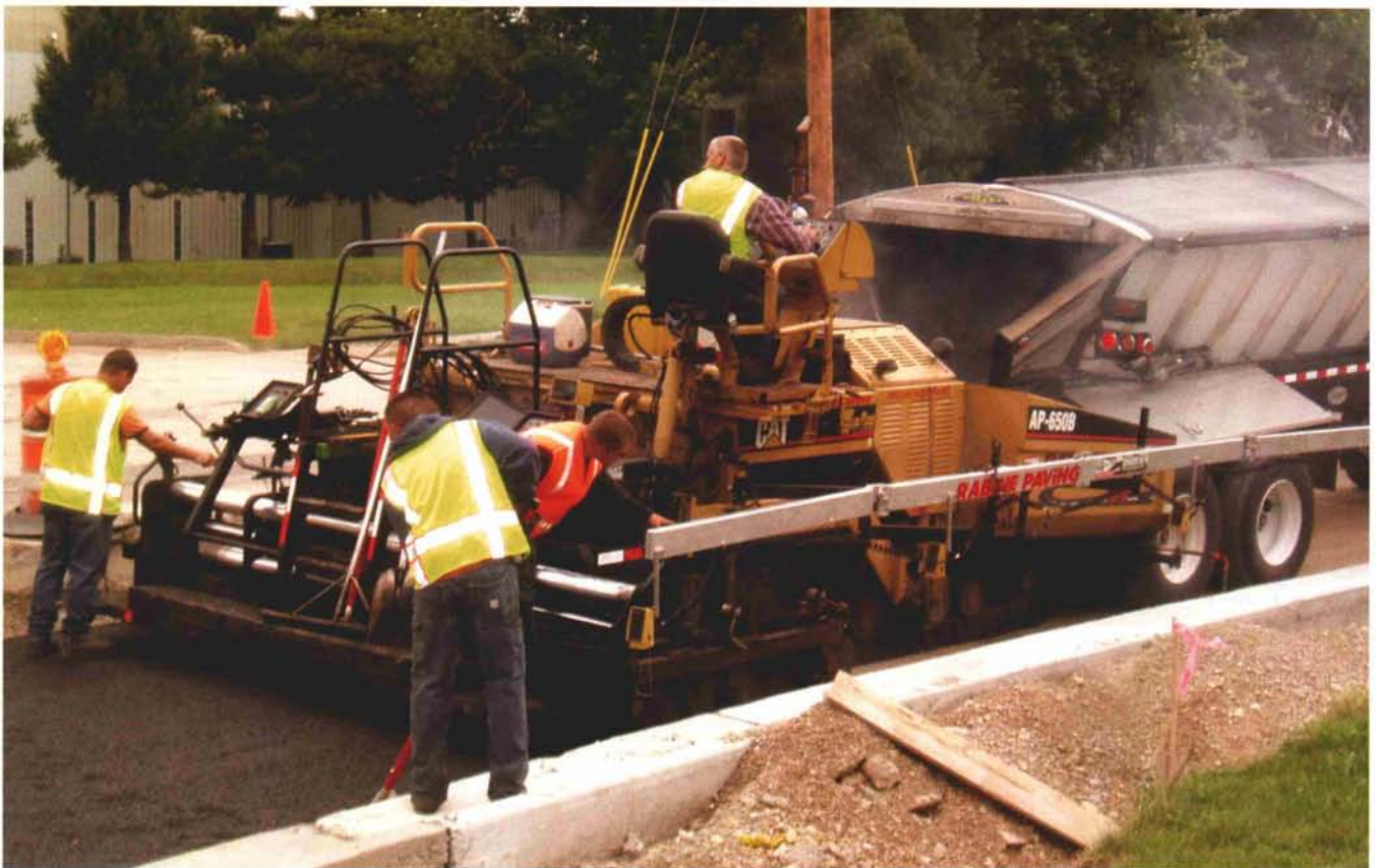
Caterpillar highway/road paver with laser-grade control system.
