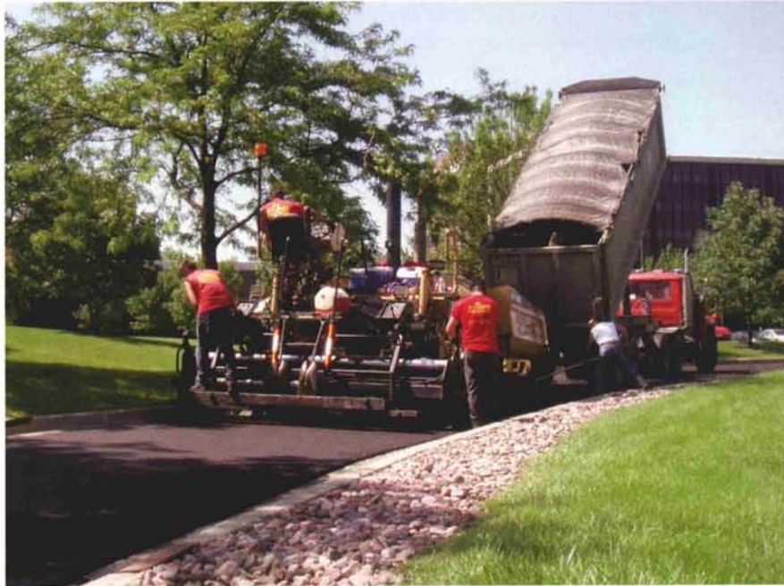
Constructing a roadway at Motorola complex in Schaumburg, IL.
