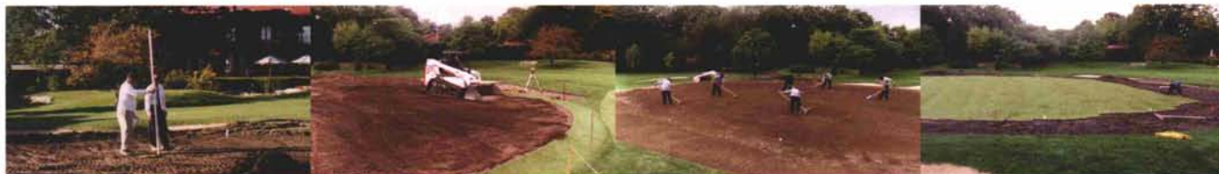
(L to R) Superintendent Bob Lively and architect Dave Esler checking grade elevations; final grading and compaction with excavator and machine; Flossmoor grounds crew doing final raking before sod work; sod being put down exactly the way it came off.
