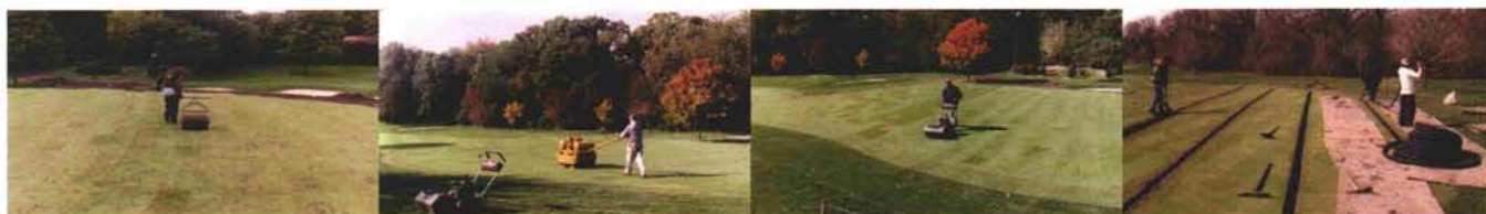
(L to R) First rolling after laying sod; second rolling one week later; first mowing 10 days after sodding; TDI installing drain lines in spring 2004.
