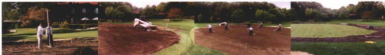
(L to R) Superintendent Bob Lively and architect Dave Esler checking grade elevations; final grading and compaction with excavator and machine; Flossmoor grounds crew doing final raking before sod work; sod being put down exactly the way it came off.
