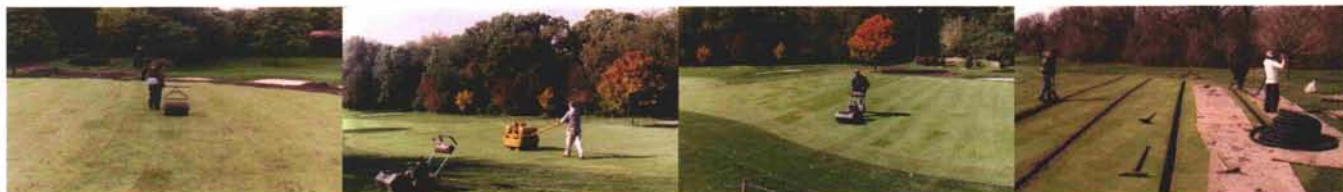
(L to R) First rolling after laying sod; second rolling one week later; first mowing 10 days after sodding; TDI installing drain lines in spring 2004.
