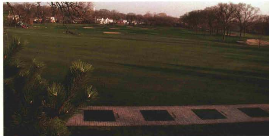
New one-acre range tee built with internal drainage every 20 feet and USGA root zone. All-weather tee mats were inlaid into rustic paving brick; renovated range also included new, enhanced target greens.
