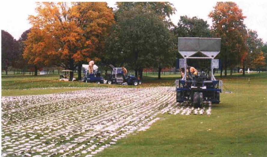
Drill-and-fill machines in action.
