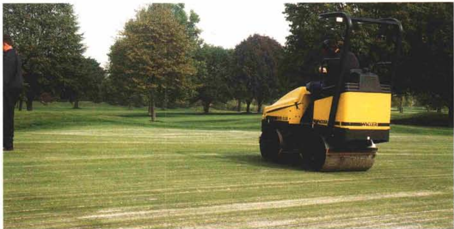
One-and-a-half-ton vibratory roller.
