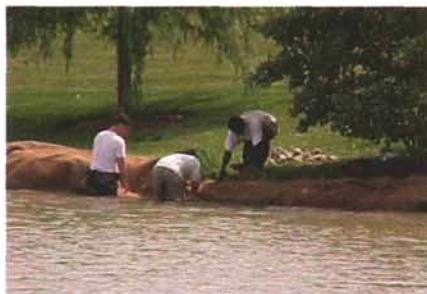
Shoreline repairs for erosion control are very important in conservation of soils.
