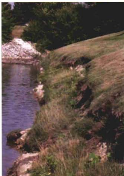
Images 4 & 5: Weed growth and/or slope erosion can degrade the appearance of conventional detention basins.
