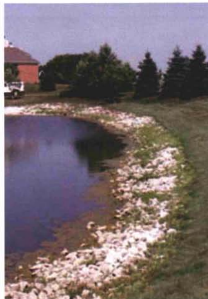
Images 4 & 5: Weed growth and/or slope erosion can degrade the appearance of conventional detention basins.
