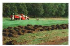
Grading of the surrounding banks also took place. Areas that settled from where trees had been removed were filled with topsoil and brought up to grade. Central Sod Farms provided Penncross bentgrass sod in big rolls. Straight bluegrass sod was used on the banks and rough. In good weather, two tees a week could be completed.
