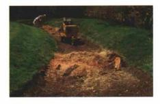
After the excavation, approximately seven inches of sand was placed within the bunker and compacted. The sand originally used in the bunkers was Reliable sand. That sand is no longer available. C9 sand, which most closely resembles the original sand, continues to be used in the bunkers. This sand drains relatively well and becomes very firm over time, although it is a little coarser than most bunker sands that are commonly used.
