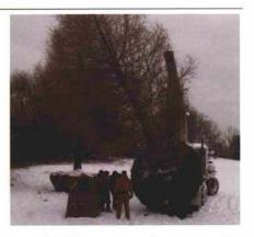
Bunker restoration was relatively simple as bunkers that were either filled in or allowed to grow over still maintained their original shape. The outlines were painted and the bunker cavity was excavated. Seth Raynor, in his 1922 renovation, installed an extensive drainage system throughout the golf course, including all of the bunkers. Because of this, additional drainage was not required.
