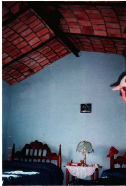
My "techos," showing the bedroom and the arched ceiling of bricks.
