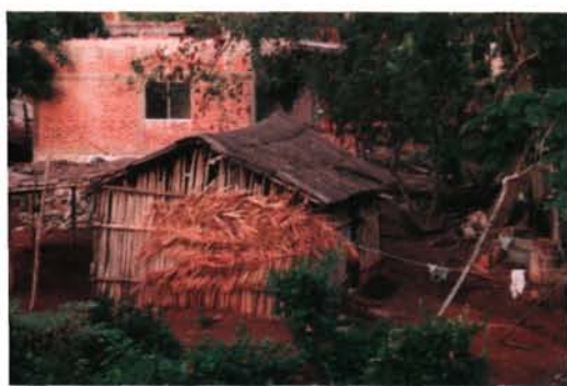
This is a typical home HfH is trying to replace.
