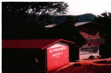
The library (biblioteca) and primary school in Chacala, Mexico.
