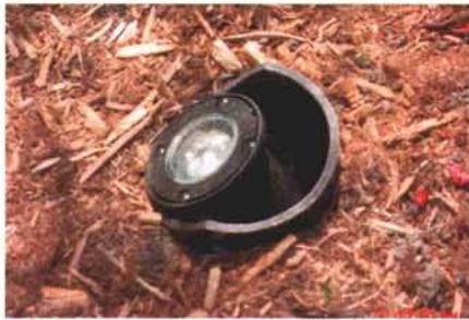
This is an adjustable ground-installed light. It would be used for lighting signs, walls, etc.
