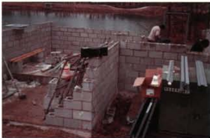
Shoreacres' building goes up around existing transformer.
