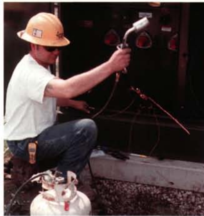
Working on the transformer at CGC.
