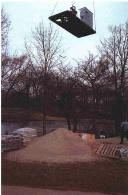
Lifting pump station into pump building at Shoreacres.
