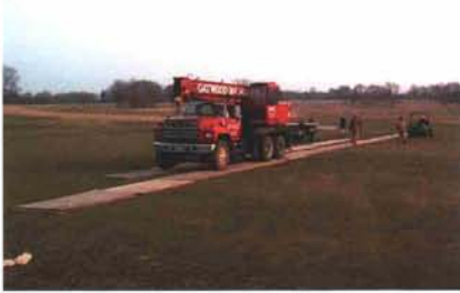
Truck traveling across plywood at CGC.
