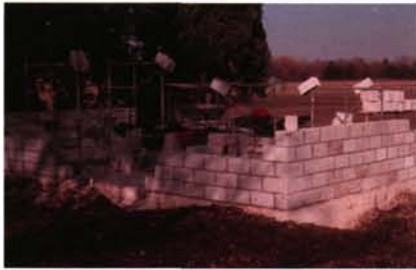
Erecting building at CGC.
