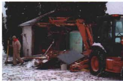
Demolition of old pump station at CGC.
