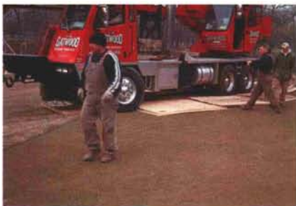
Crane on no. 18 at Shoreacres.
