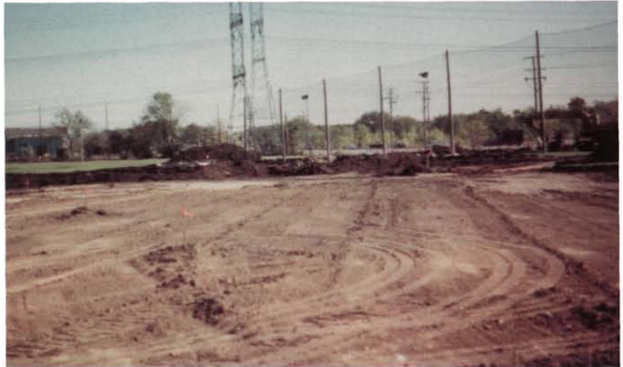
Site preparation in advance of dome construction at Salt Creek.
