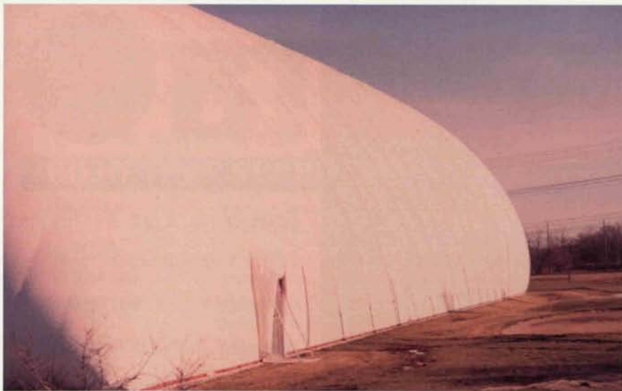
Exterior shot of the Salt Creek dome.
