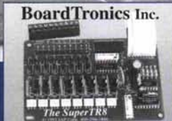
CONTROLLER BOARD REPAIRS
