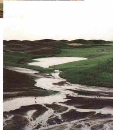
7/25/93—Lost time, lost materials and washouts remain after 'catastrophic' rains.
