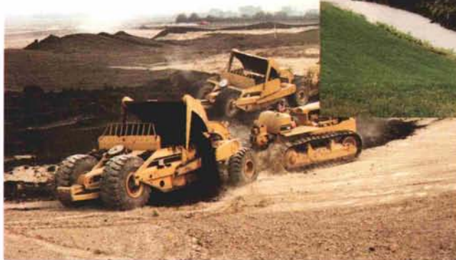
5/22/92—Noise and dust fill the air as Cat Panscrapers respread topsoil.
