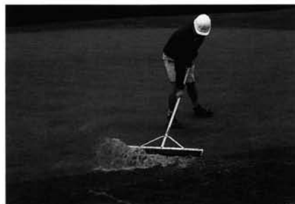
Standing water on greens that requires squeegeeing following heavy rainfall is an obvious sign of poor surface drainage.
