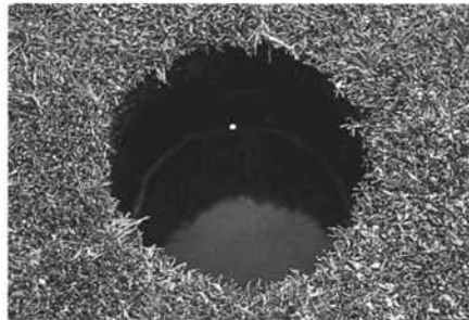
Standing water in the hole after a green has been deep-tine-aerified is a clear indication of poor subsurface drainage and the need to rebuild.
