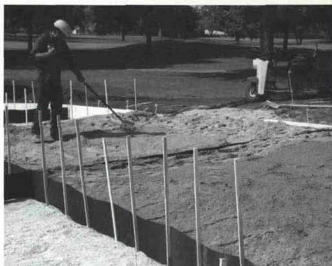
All of the various rootzone cells are backfilled by hand.
