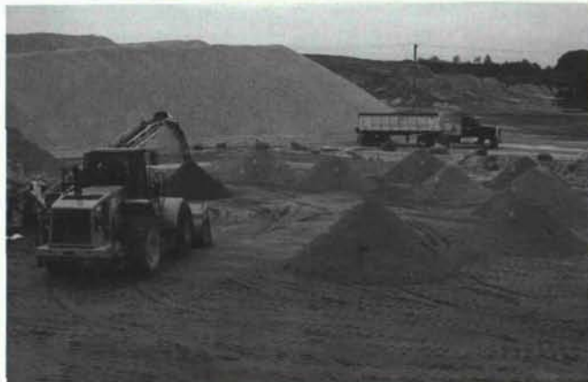
Off-site mixing for the green rootzones mixes at the Feltes Sand & Gravel Co.
