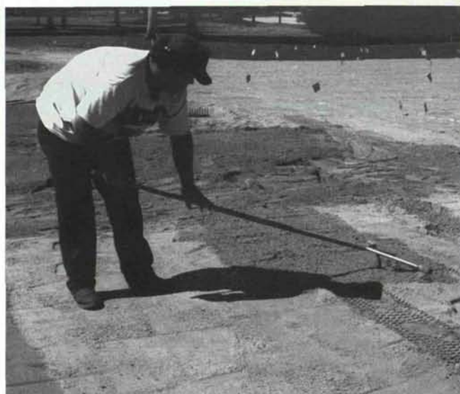
All work is done by hand to prevent cross contamination of soil mixes.
