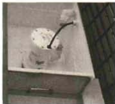
Computerized pump system keeps fluids within 1/4 inch depth, stainless steel removable screens filter large debris.
