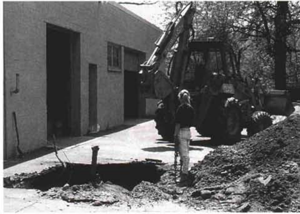
First process of digging hole to pull 1,000-gallon heating oil tank.
