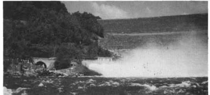
Summerville Dan with 3 tubes putting out 2,600 cubic feet a second of white water.
