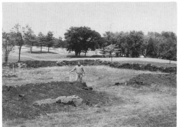
Tony setting grade stakes for the new experimental green.
