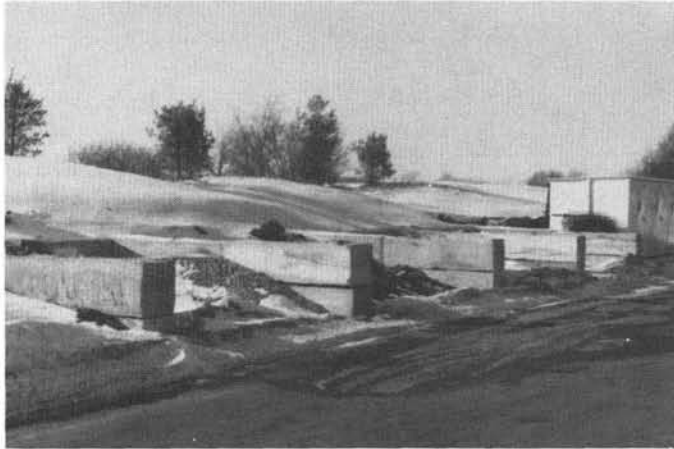
Cantigny G.C. Storage Bins
