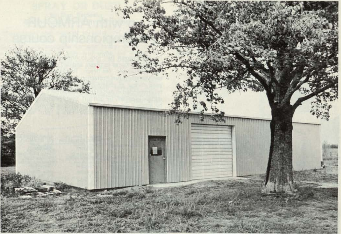
The Illinois Turfgrass Foundation provided funds for this 40' x 60' building on the turf research area at Urbana. The building, when completed, will provide space for equipment and chemical storage as well as a field laboratory. The field plot area at Urbana has been doubled so that more applied research can be done.
