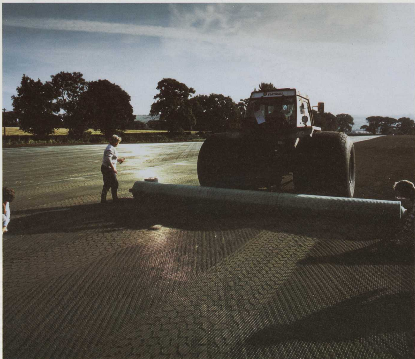
SODNET being laid on Lindum turf fields.
